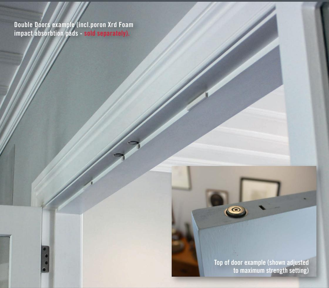
Top of door example (shown adjusted to maximum strength setting)
